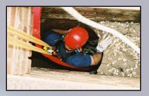
The term "confined space" can be used to describe a wide variety of work areas – underground utility vaults, storage containers, manholes, HVAC units, and ice resurfacer snow melt pits. Any space that is large enough to enter but not designed for continuous occupancy falls under the category of a confined space.
