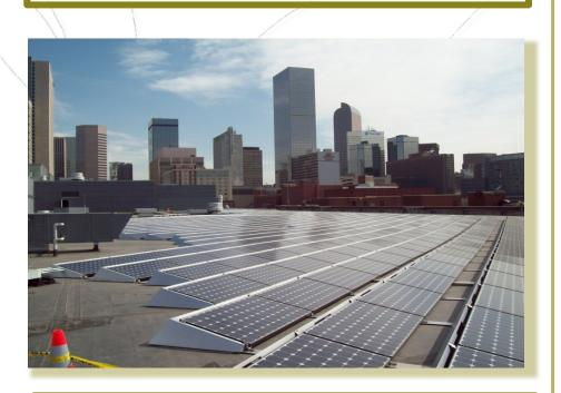
The roof of the Colorado Convention Center hosts a 301kW solar array system to take advantage of the Colorado sunshine and convert it to energy for our building. <u>CLICK HERE</u> to see what the system is currently producing.
