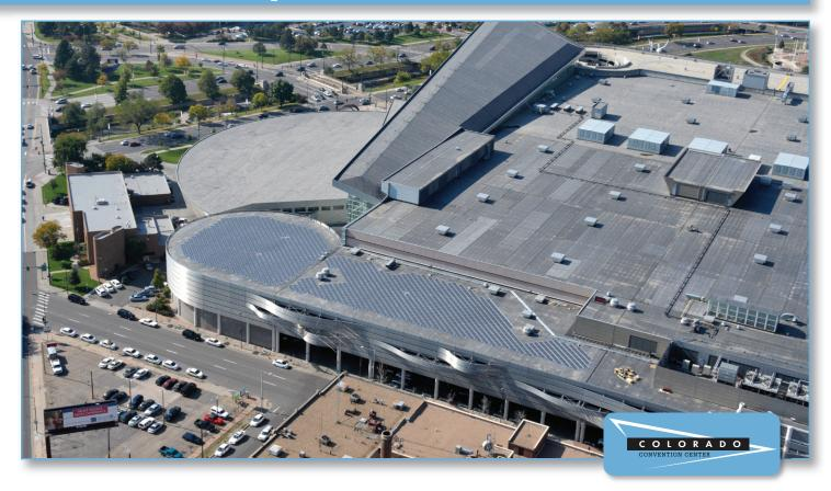
The Colorado Convention Center is a state-of-the-art facility in the heart of exciting downtown Denver. The convention center is now hosting a landmark renewable energy project, a 300 kilowatt solar power system. Covering 30,000 square feet atop the convention center, this solar array demonstrates Denver's commitment to environmental sustainability.
